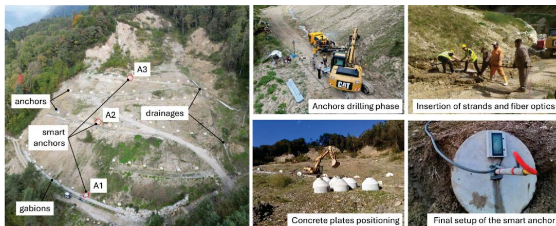
Fig. 3 Site overview with installed anchors, drilling and anchors installation, followed by fiber optic placement and setup
