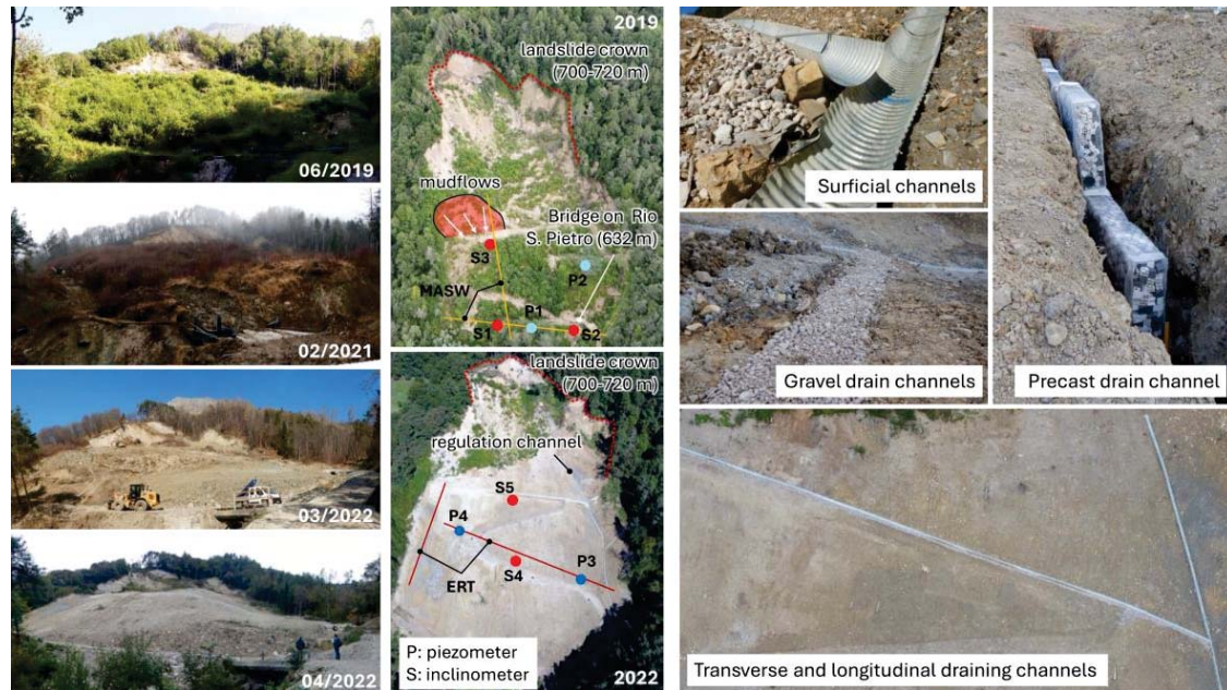
Fig. 2 First phases interventions: reshape and drainage system realization
