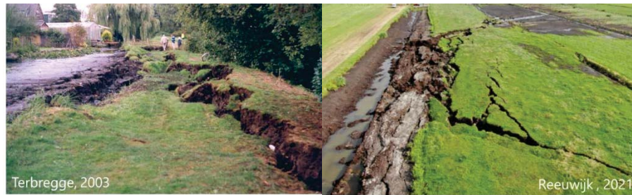
Fig. 1. Left: The dike breach at Terbregge, The Netherlands, in 2003. Right: the dike breach at Reeuwijk, The Netherlands, in 2021. In both cases, the canal is on the left side and the polder is on the right side. The canals were rather shallow and up to about one meter deep, limiting the development of the breach and the water that could flow into the polder.
