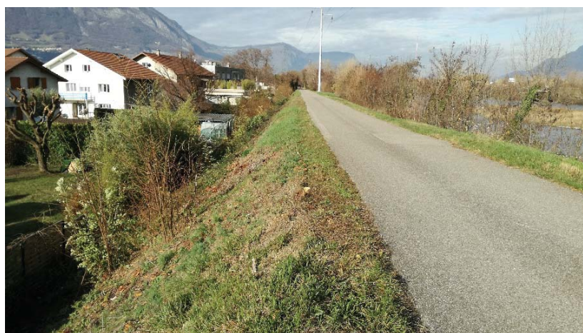
Figure 1. Embankment along the Drac River
