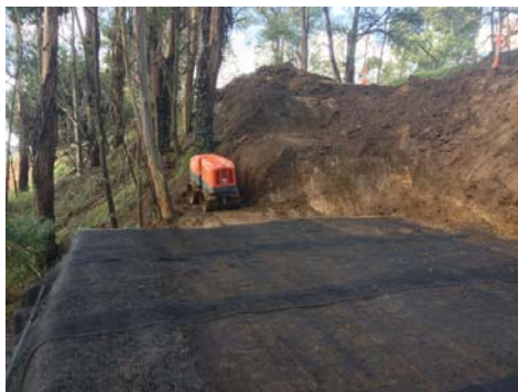
Figure 3. General construction process of geogrid-reinforced soil zone
