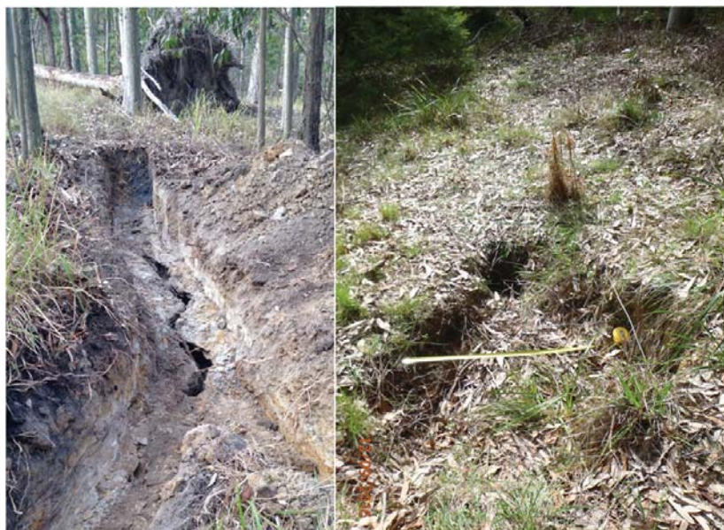
Figure 1. Examples of exposed bedrock crack and hole at Rhondda in 2016
