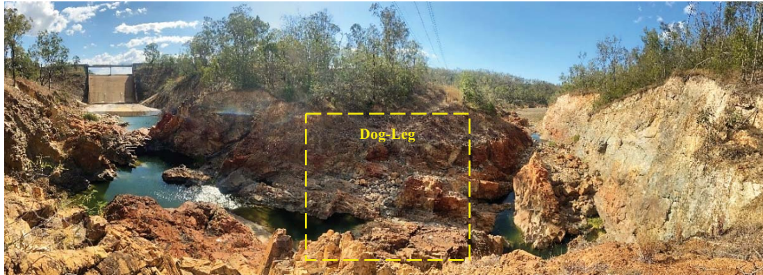
Figure 1. Spillway Return Channel general overview from the “Dog-Leg”
