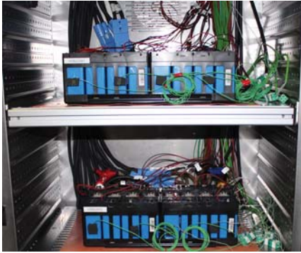
Fig. 3. Contacted battery modules in the climate chamber
