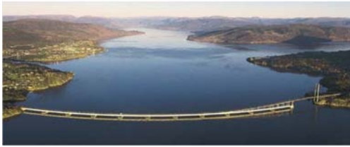
Fig. 1. The Nordhordland bridge as seen from south-southwest. The floating part can be seen as the white beam resting on the pontoons. (Photo: Helge Sunde)
