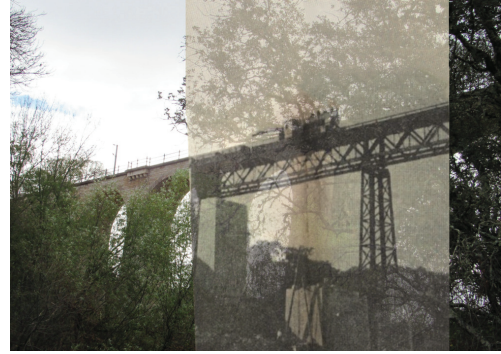
Fig. 1. Composition of the actual Quinta Nova bridge in September 2023 and its construction process during June 1933, showcasing the original metallic structure in the background. Adapted from (Costa, 1934).
