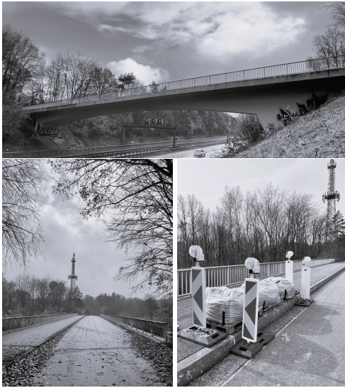
Fig. 1. Vahrendorfer Stadtweg bridge view from north (top) and northeast (bottom left), and three additional masses at the middle of the bridge (bottom right).
