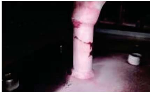
Fig. 2 Crack of the jig
