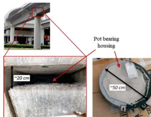
Fig. 1 Pot bearing housings in railway viaducts
