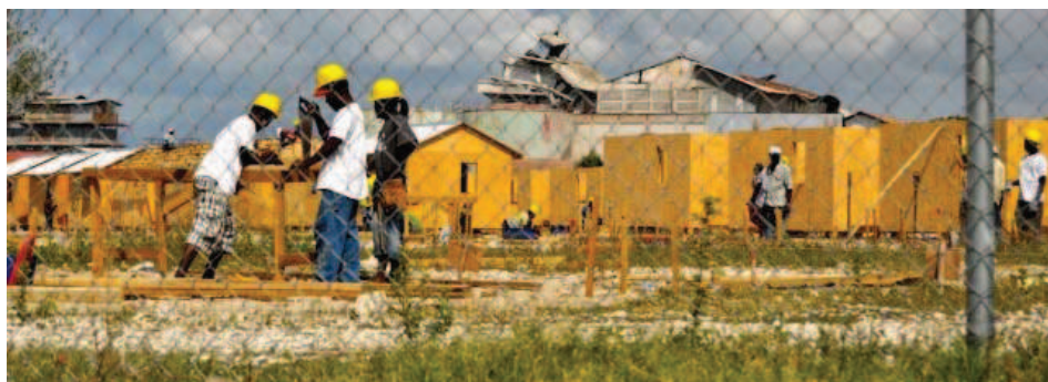
Figure 1 T-shelters under construction, Port-au-Prince. Photo: Anshu Sharma
