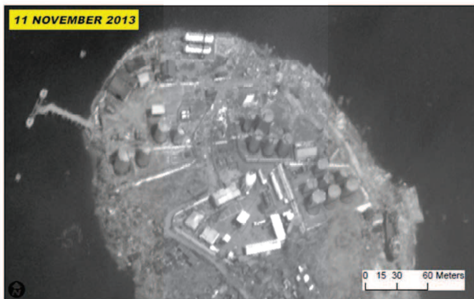
Figure 5 Satellite imagery of damaged industrial facility in Tacloban (credit: UNOSAT).
