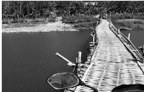
Figure 2 Bamboo bridge rebuilt using gotongroyong in desa Seloharjo.
