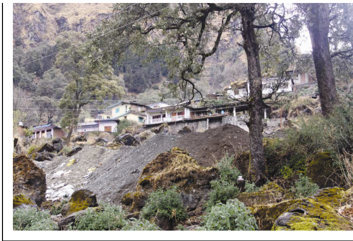
Figure 3 Disposal of excavated debris along the hill slope in Nainital. Obliteration of surface drains by site development works for construction.
