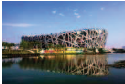
Figure 4. National Stadium 'Bird's nest' Beijing
