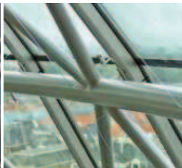
Figure 2. Smooth connection of tubes
