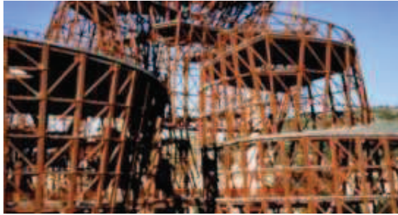
Figure 12. Load bearing structure of Guggenheim Bilbao during construction phase
