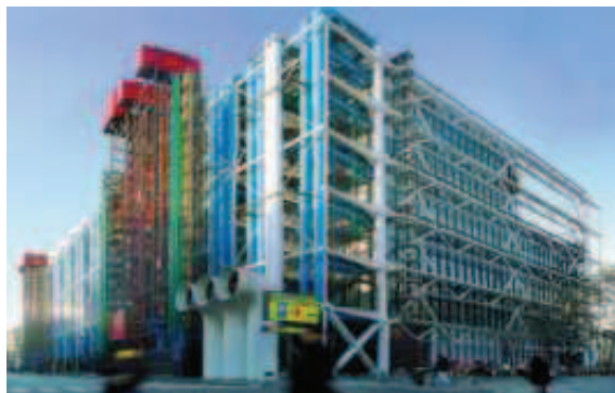
Figure 6. Centre Pompidou, Paris
