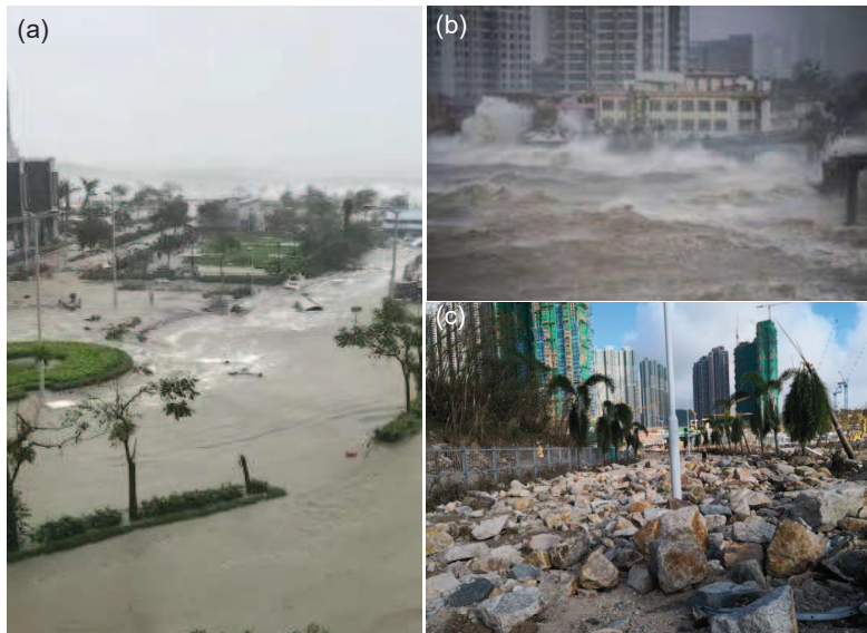
Figure 2. Damage to the urban areas of Hong Kong by Typhoon Mangkhut in Sept. 2018: (a) flooding of South Tseung Kwan O; (b) wave impact on the shoreline at Heng Fa Chuen; (c) street covered by fill materials washed away from seawall.
