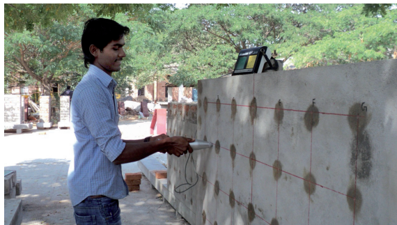
Fig. 23 Rebound hammer data collection on a finished brick wall
