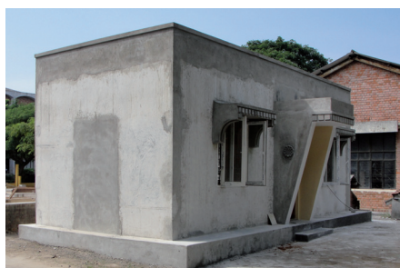
Demo building before colour washing
