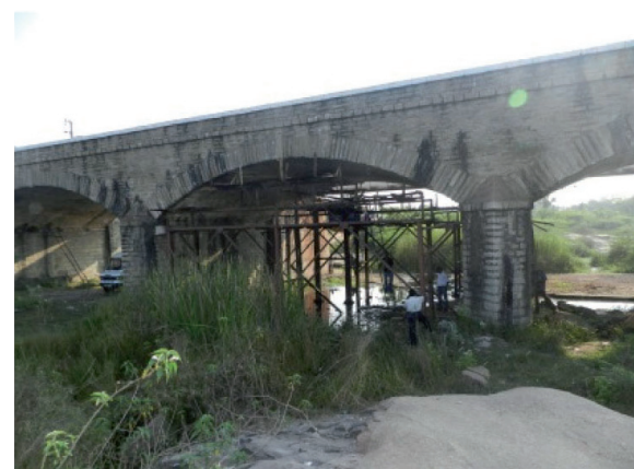
Fig. 2 Wireless sensors instrumented in a stone arch bridge along with conventional sensors
