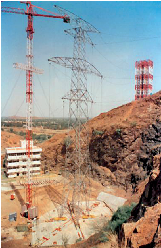
An aerial view of the TTRS facilities
