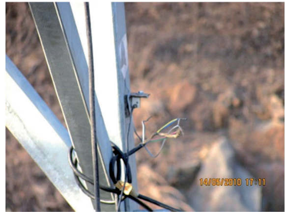
Fig. 3 Location of accelerometer and strain gauges in the experimental tower
