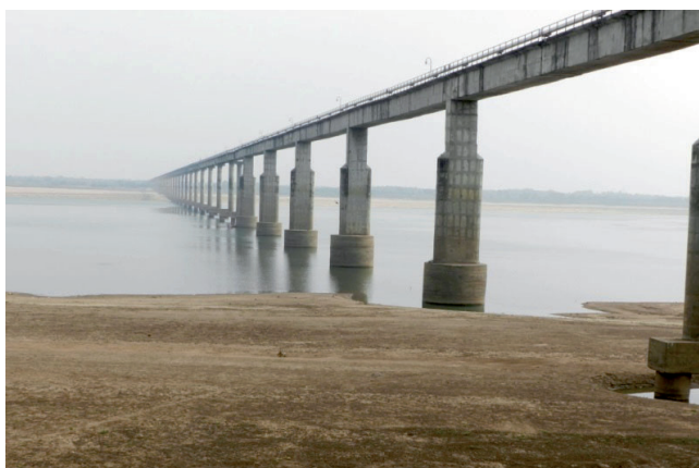
Bridge across River Godavari carrying HPCL and GAIL Pipeline
