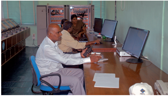
Control room of TTRS
