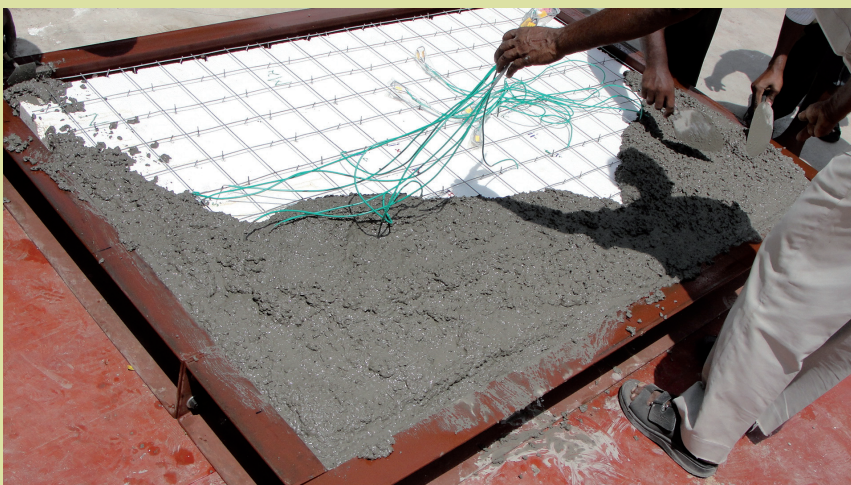
Casting of EPS test specimens
