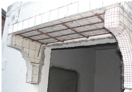
Window lintel using EPS
