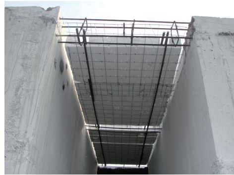
EPS roof panel for connecting two units
