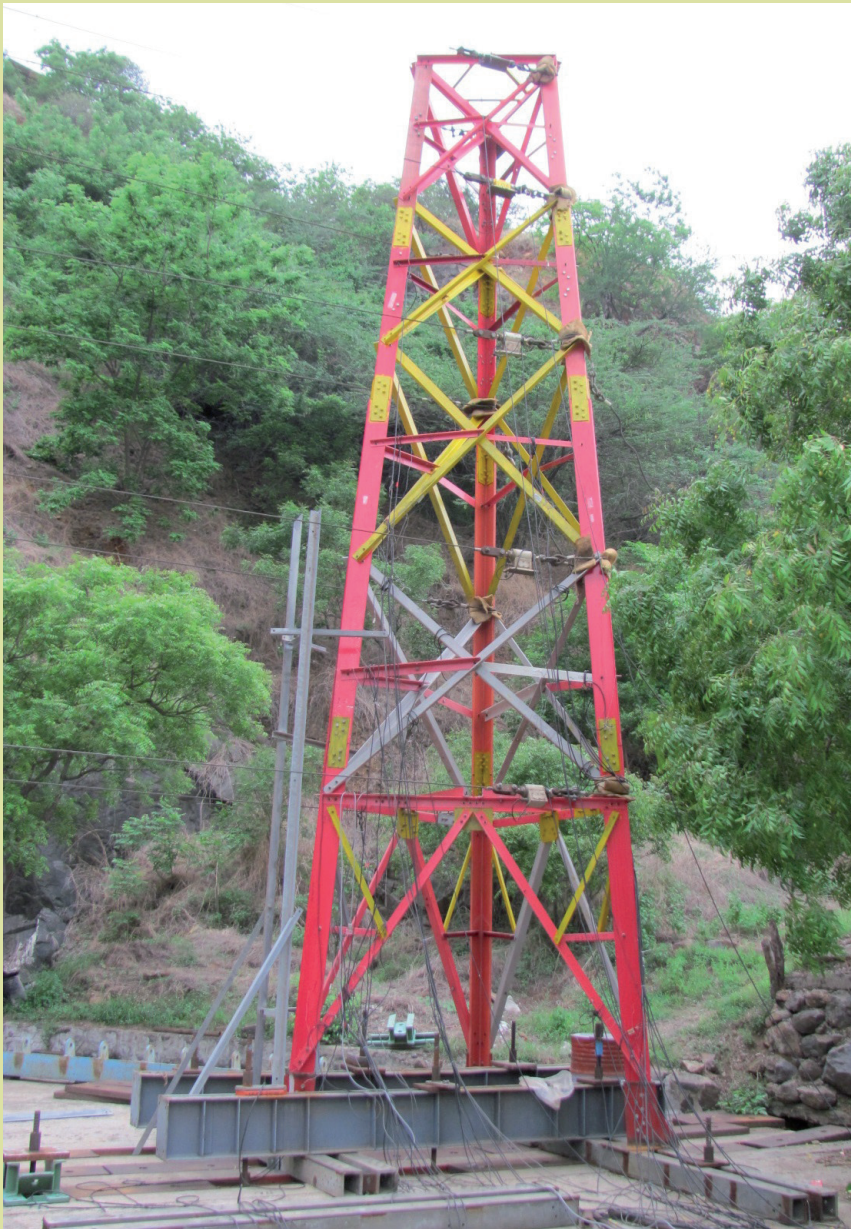
Steel-GFRP 9 m high hybrid rooftop microwave tower during test
