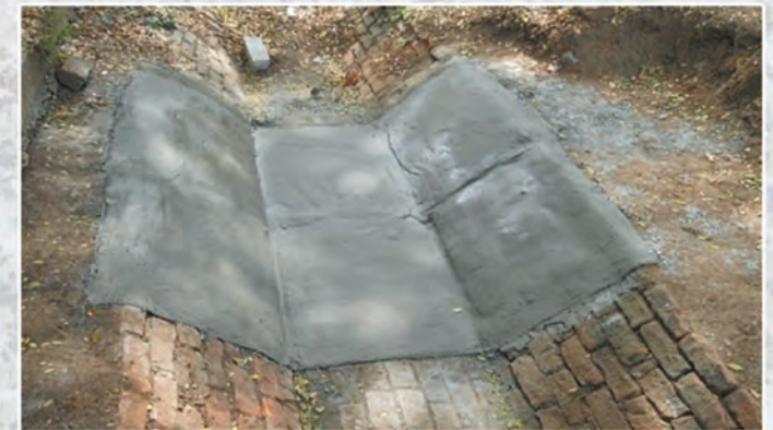
Lining of existing damaged canal using FABcrete produced through TRCPT
