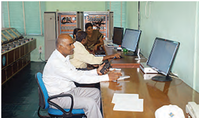
Control room of TTRS
