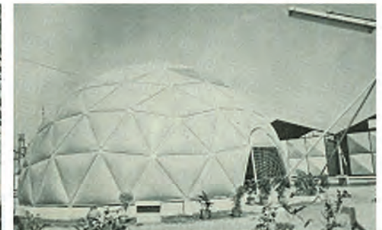
Braced dome of aluminium with glass fibre reinforced polyester cladding unit at the Indian International Trade and Industries Fair Madras, 1968 - Structural Design by CSIR-SERC.
