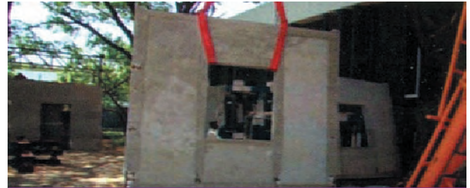
Wall Panel with window opening being shifted
