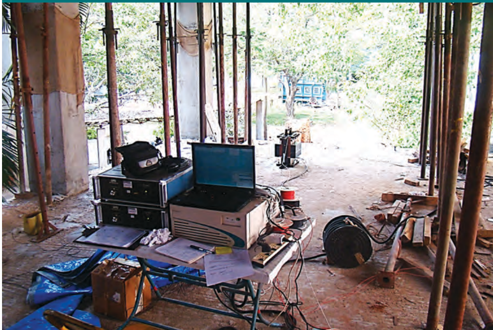
Measurement of vibration excitation of Experimental Link Building of CSIR-SERC with APS 400 electro dynamic shaker in vertical mode
