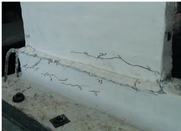
Sliding type of failure through the horizontal bed joint, at lintel level
