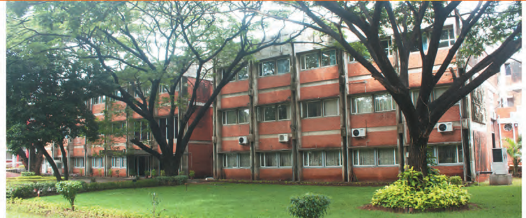
The main building of the Campus has incorporated partially prestressed concrete beams produced at the casting yard
