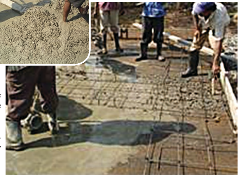
A view of construction of High Volume Flyash Concrete White topping at CSIR-SERC
