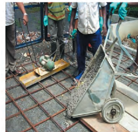
Laying of GPCC
