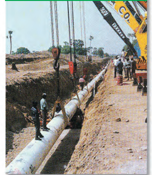
Strain monitoring of the HBJ gas pipeline during lowering
