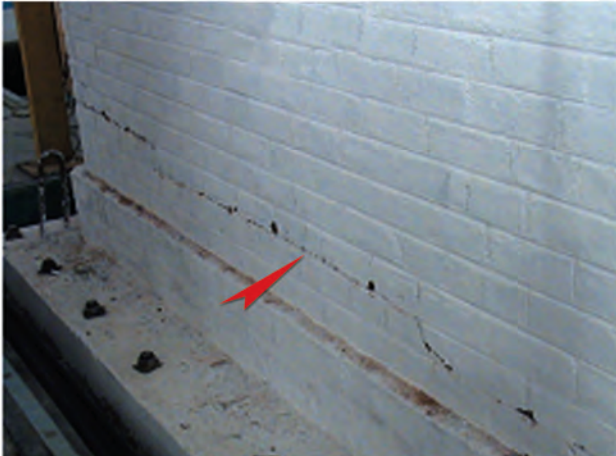
Sliding type of failure through the horizontal bed joint, at plinth level - View 1
