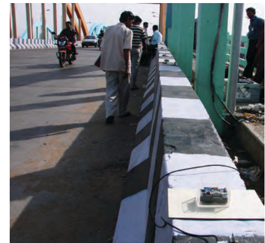
Field demonstration of SHM using WSSN at Velachery-Tambaram bridge, Chennai.
