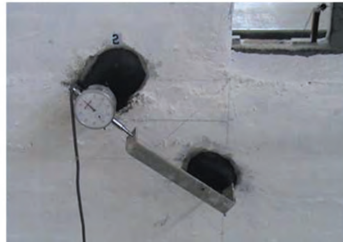
Strain gauge-based sensor system for measuring the crack opening
