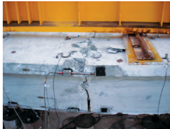
Specimen at failure load
