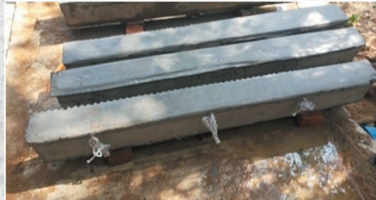
Strengthening of beams
