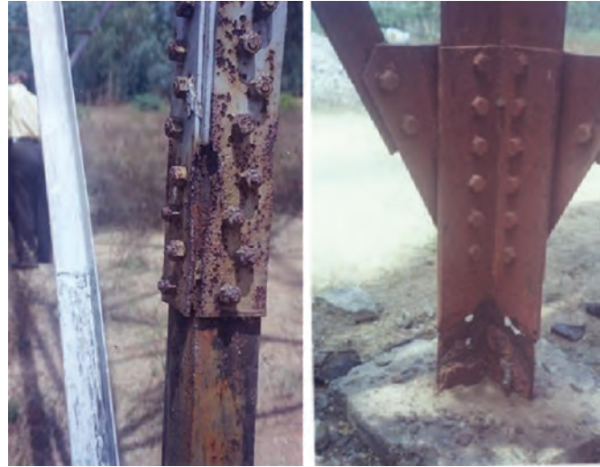
Corrosion of tower leg member
