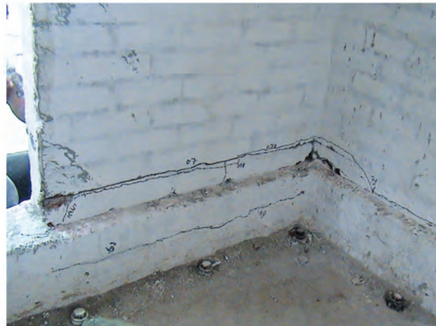
Sliding type of failure through the horizontal bed joint, at plinth level - View 2
