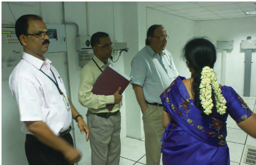
DG at Data Centre
