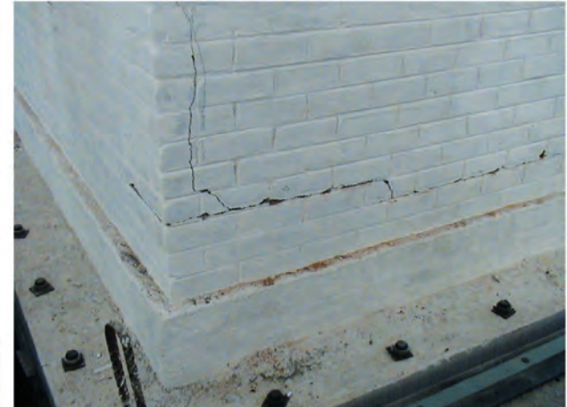
Corner separation due to out-of-plane bending
